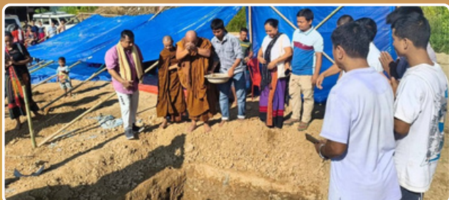
Bhoomi Pujan of School building construction of Kalindi Rani Vidya Mandir in Mizoram
